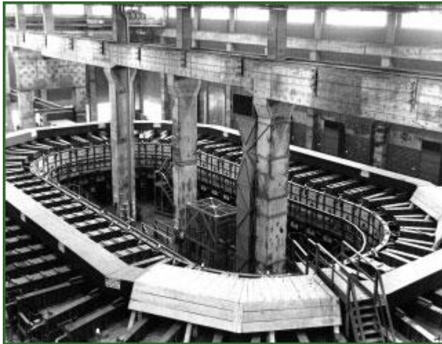
Alpha Racetrack, Y-12 Electromagnetic Plant, Oak Ridge
